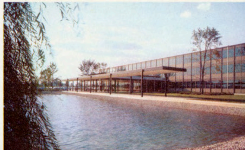
South facade of Research Building.
